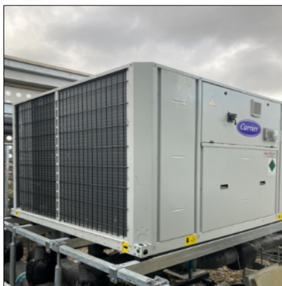
Caption: Battery storage installed through Public Sector Decarbonisation Scheme Phase 1.
